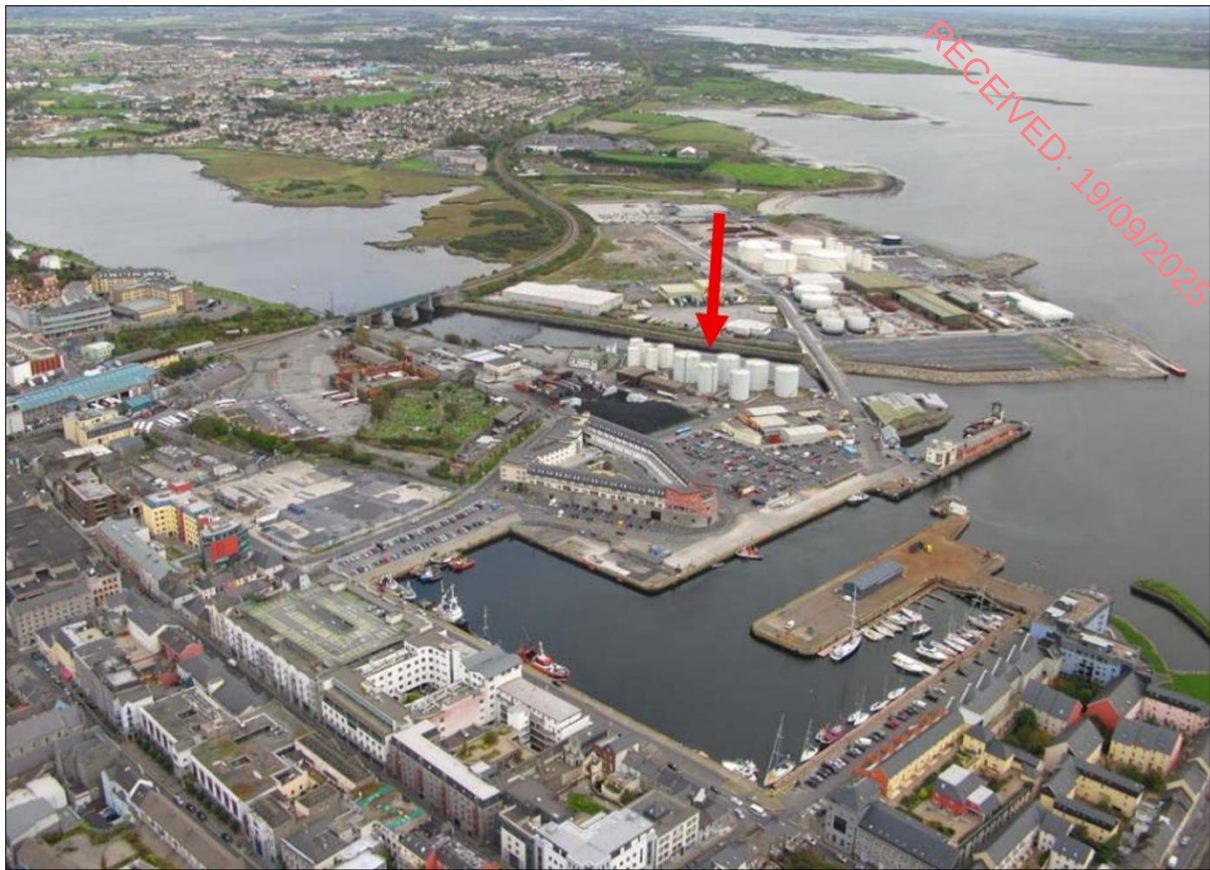
Figure 14-13 Aerial image of the port, showing the fuel silos within the subject site (centre of photo – indicated by red arrow) prior to their removal in c.2018 (Source: Port of Galway)
