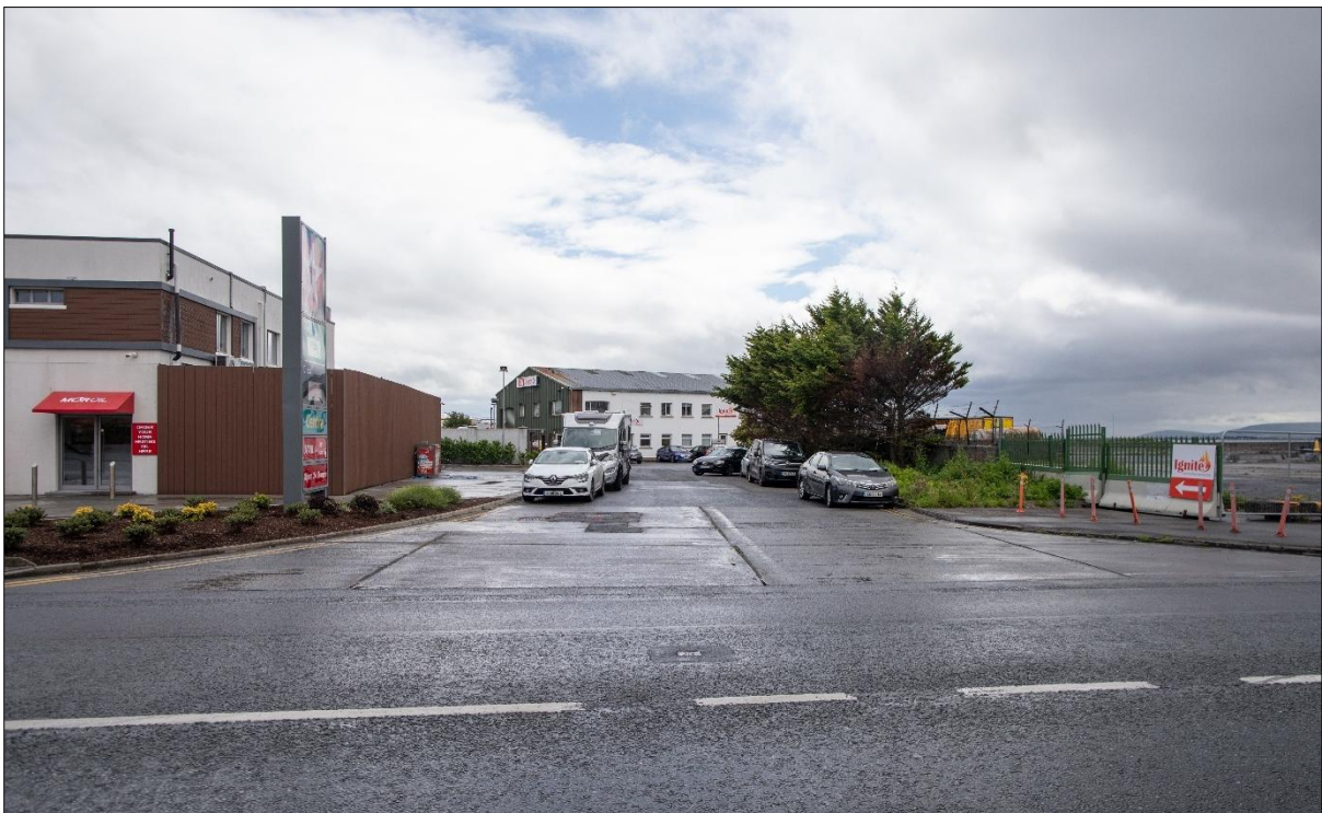
Figure 11-6 A View Towards the site from Lough Atalia Road to the North. The Two Storey Pitch Roofed Building in the Middle Distance is on the Site
