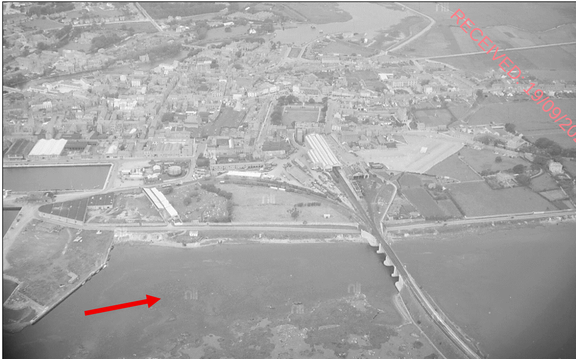
Figure 14-10 Aerial view of Galway docks, railway bridge and Forthill cemetery facing west (1954). Red arrow points to general location of subject site. Note the building on foreshore which corresponds to the building in this position on the 25-inch OS map (Source: National Library of Ireland)
